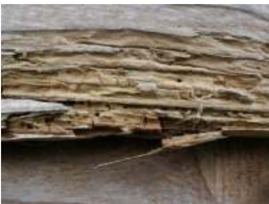
Image 0-4; Common furniture beetle damage
